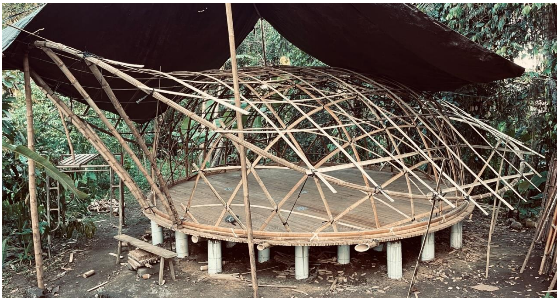
Figure 2. Completed main structure of one dormitory unit.
