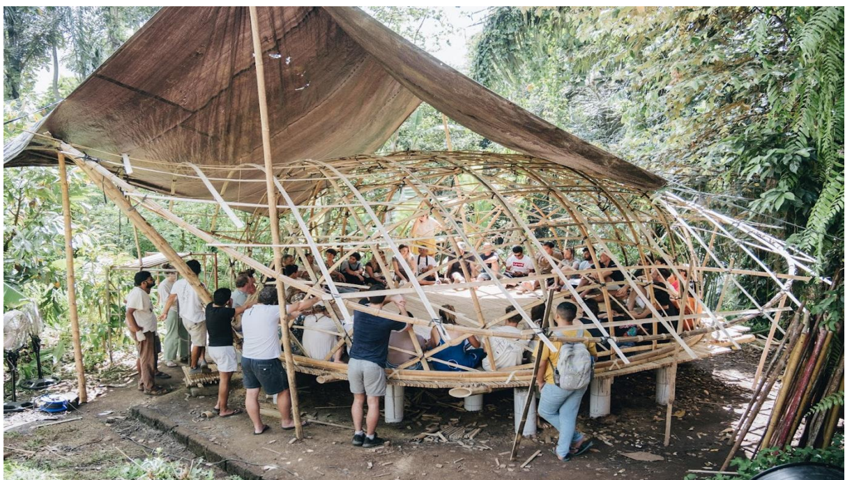
Figure 9. Workshop Team inside Grid shell structure
