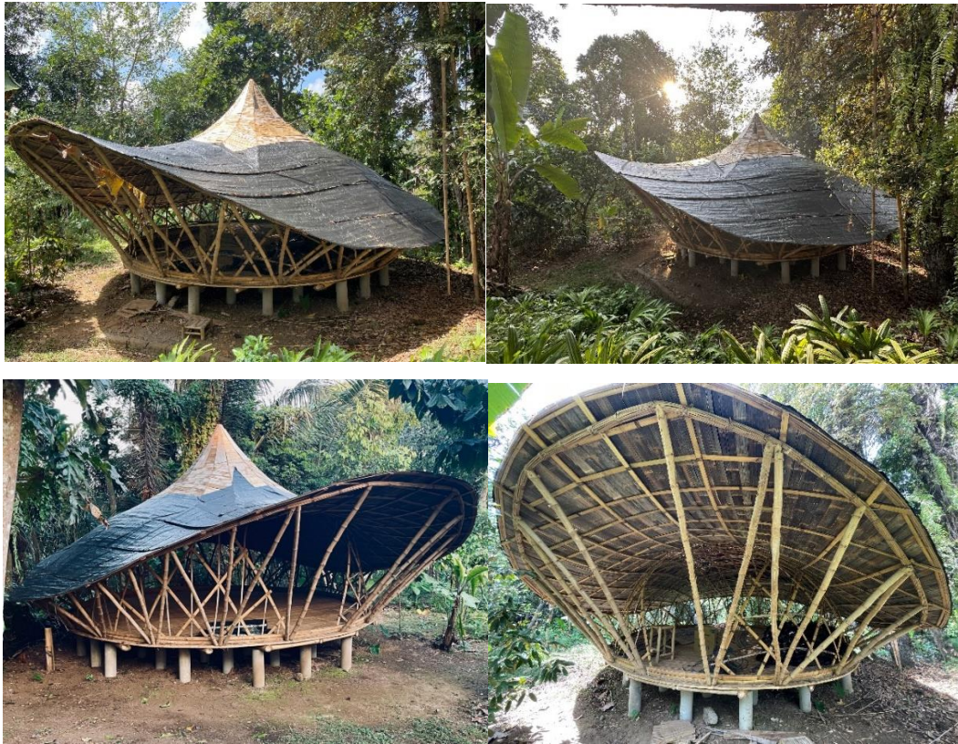
Figure 10. Current construction progress of structures
