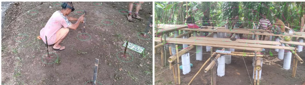
Figure 4. Labelling foundation position and installation of the floor
