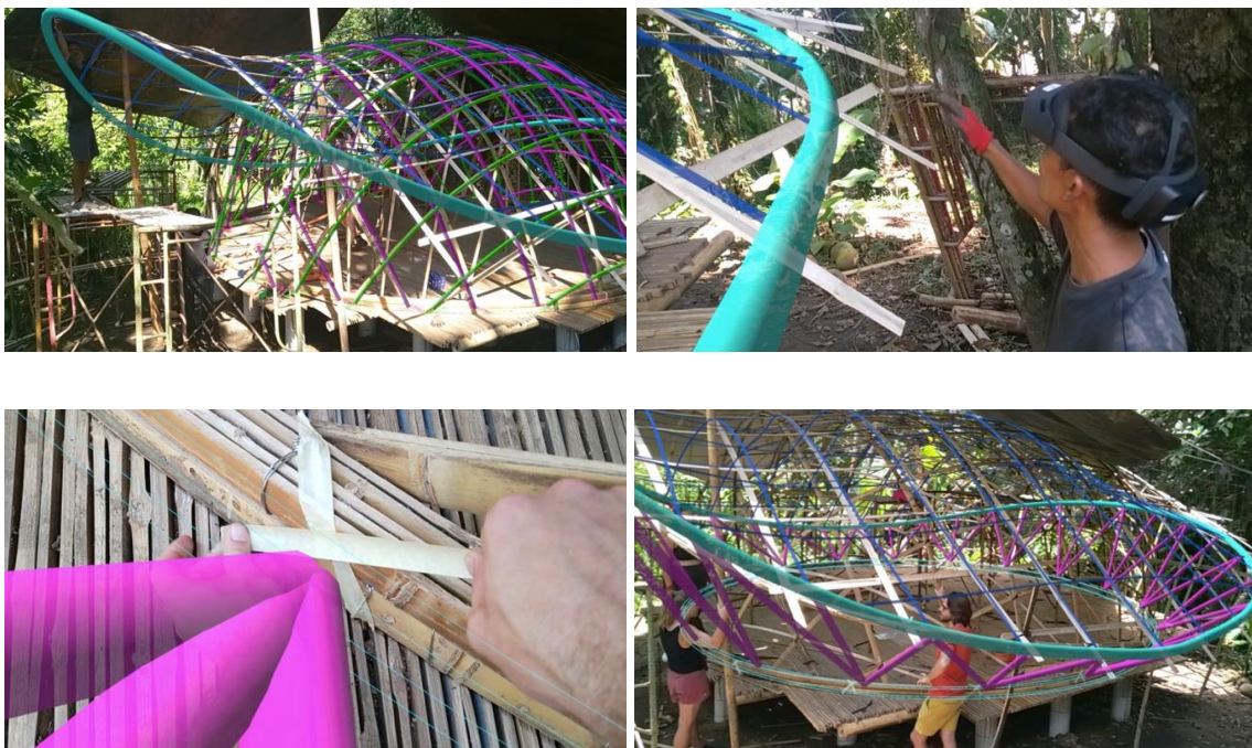
Figure 8. Installing the “Lidi Bundle” roofline
